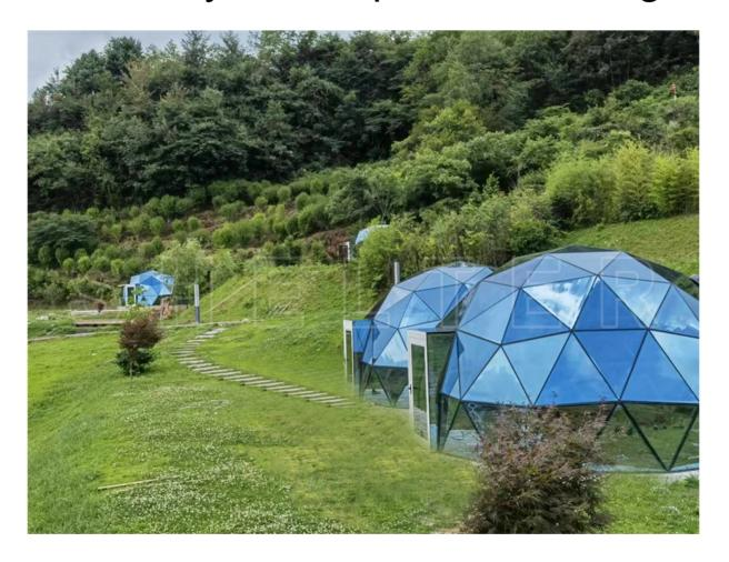
Wood platform diameter 12 m, House floor diameter 8 m, Center height: 4.0m, construction Aluminum frame, Roof: double layered laminated tempered glass (5mm tempered glass + 0.76PVB + 5mm, tempered glass) Window: 2 pcs, Entrance: 1 set of single glass door, Wind load: 150km/h, Snow load: 0.5kn/m2, 2000 liter water reservoir or permanet conect, biological sewage treatment plant, 6 KW solar electric system + wind turbin with batteries.
